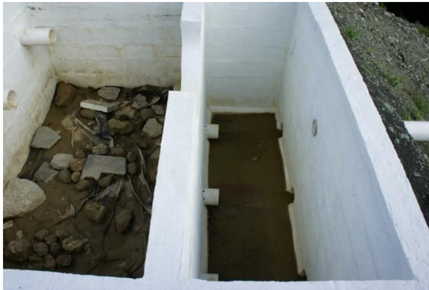
Figure 6. Detailed view of the sand filtration unit process at the new landfill. Image source: author.
