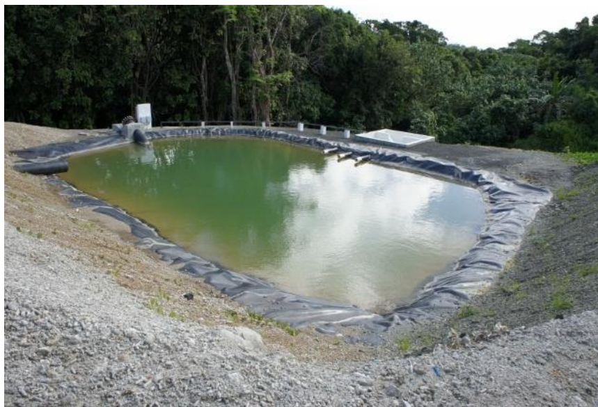
Figure 5. Leachate collection pond at the new landfill. White box on far side of pond is the sand filtration unit. Image source: author.
