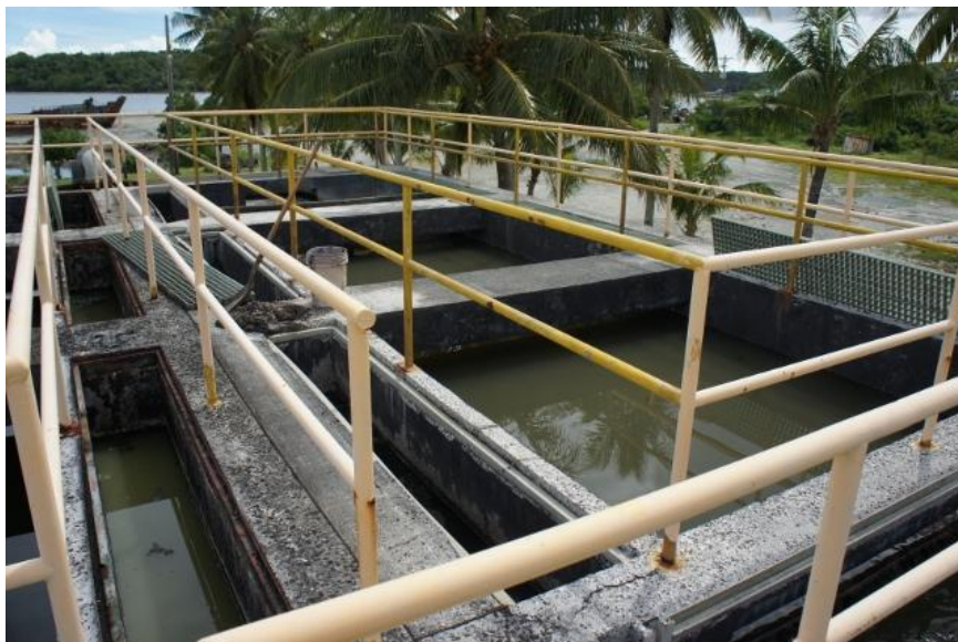
Figure 8. One flow line in the Imhoff tank sewage treatment plant. Image source: author.
