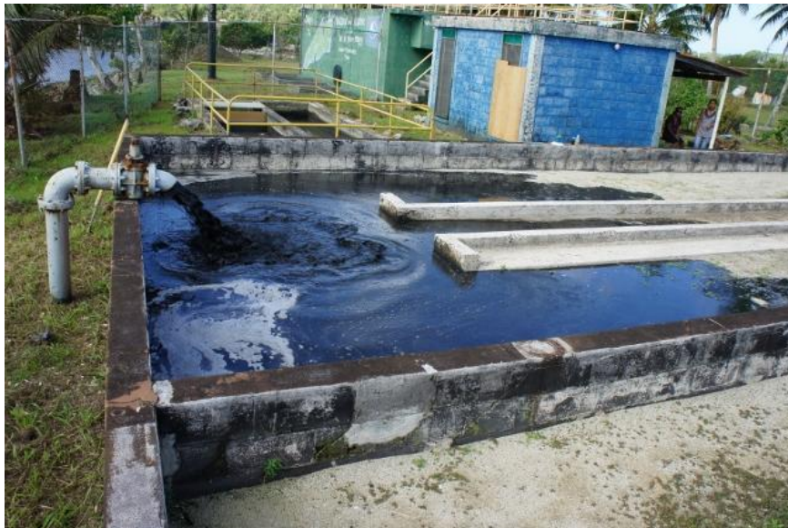
Figure 10. Sewage sludge from Imhoff tank being discharged to drying bed. Image source: author.
