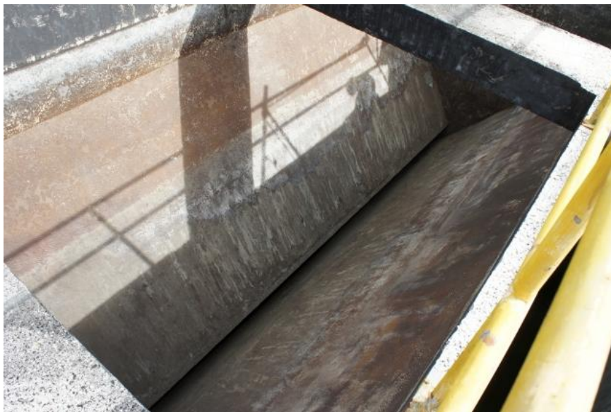
Figure 9. Imhoff tank emptied for inspection showing compartment where biocarrier matrix could be inserted. Image source: author.
