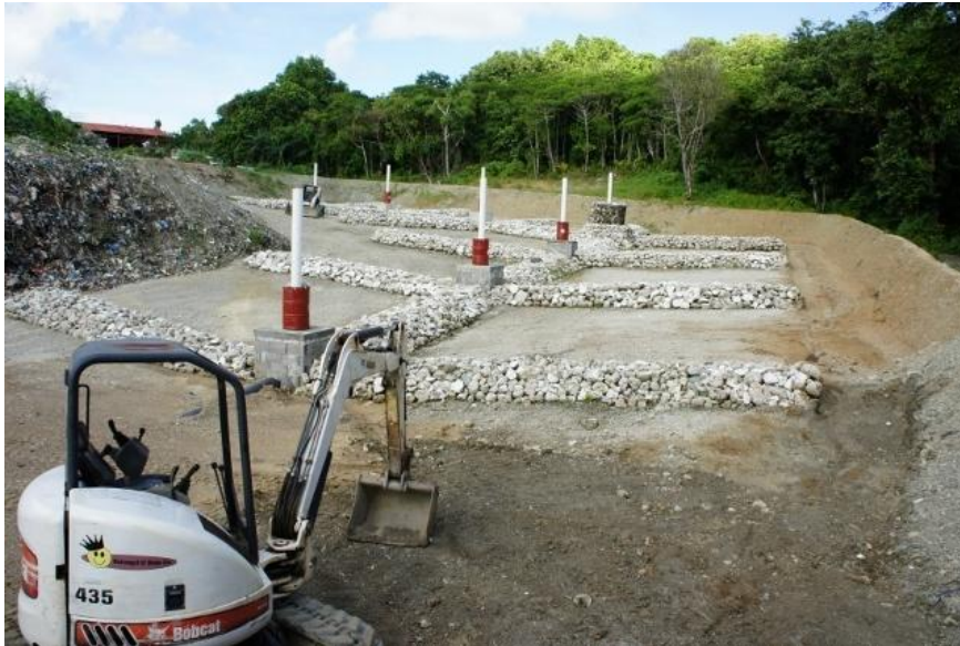
Figure 4. Newly constructed Fukuoka-type landfill on Yap prior to first use. Image source: author.
