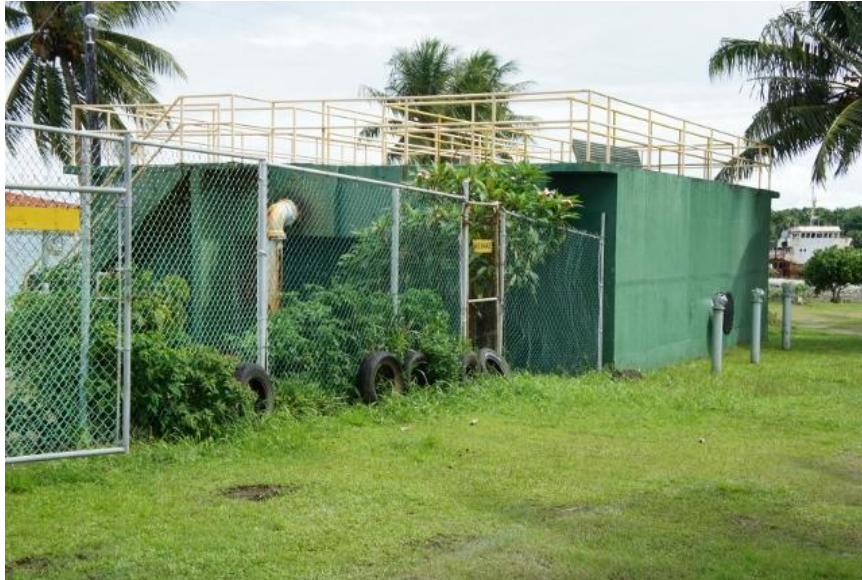
Figure 7. Imhoff tank sewage treatment plant in Colonia, Yap. Image source: author.
