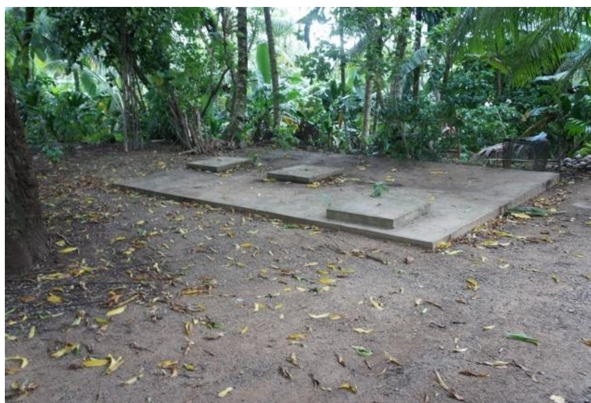
Figure 3. Large communal septic tank used in remotely located Daabach Village on Yap. Image source: author.
