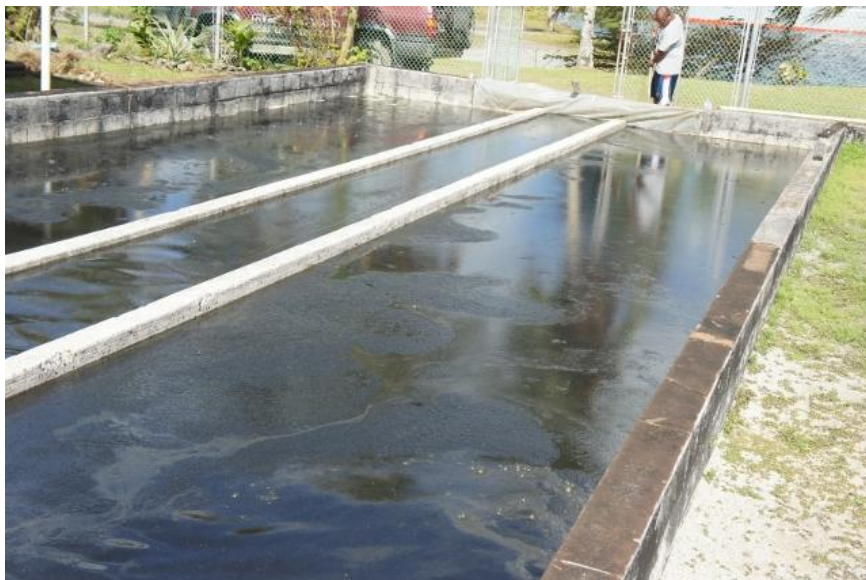
Figure 11. Fresh wet sewage sludge in drying bed at beginning of drying period. Image source: author.
