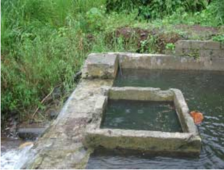
Figure 3. Pukusrik Dam, Kosrae Island
