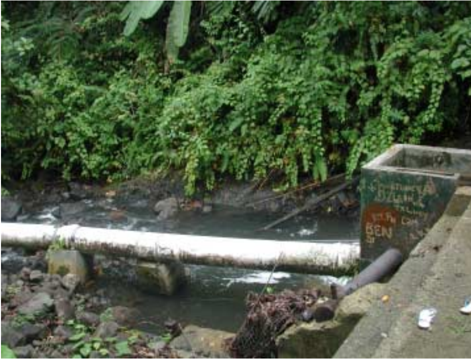
Figure 5. Malem Diversion Dam, Kosrae Island
